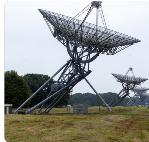
Radar & Sonar Systems
